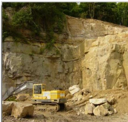
(quarrying site of stones)
